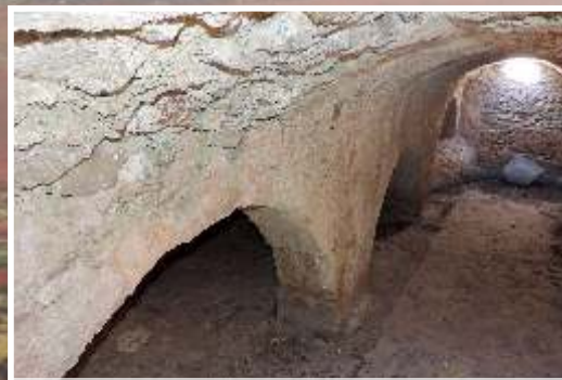
Interior of vaulted cistern
